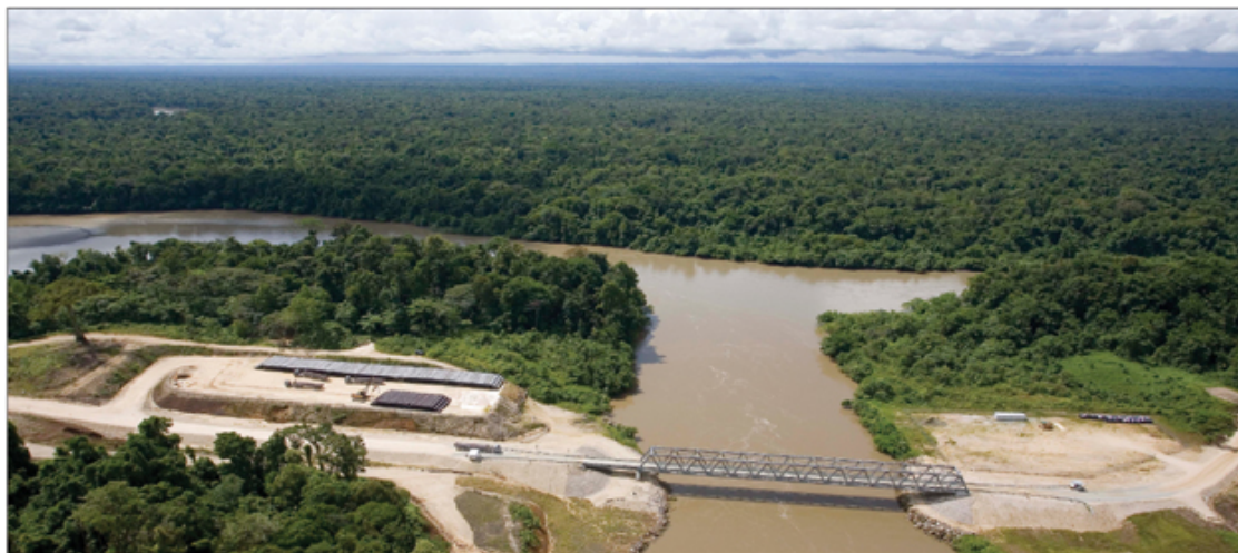
The newly constructed 435-foot Mubi River bridge is the longest of its type in Papua New Guinea and provides access from the lowlands in the south to the highlands in the north.
