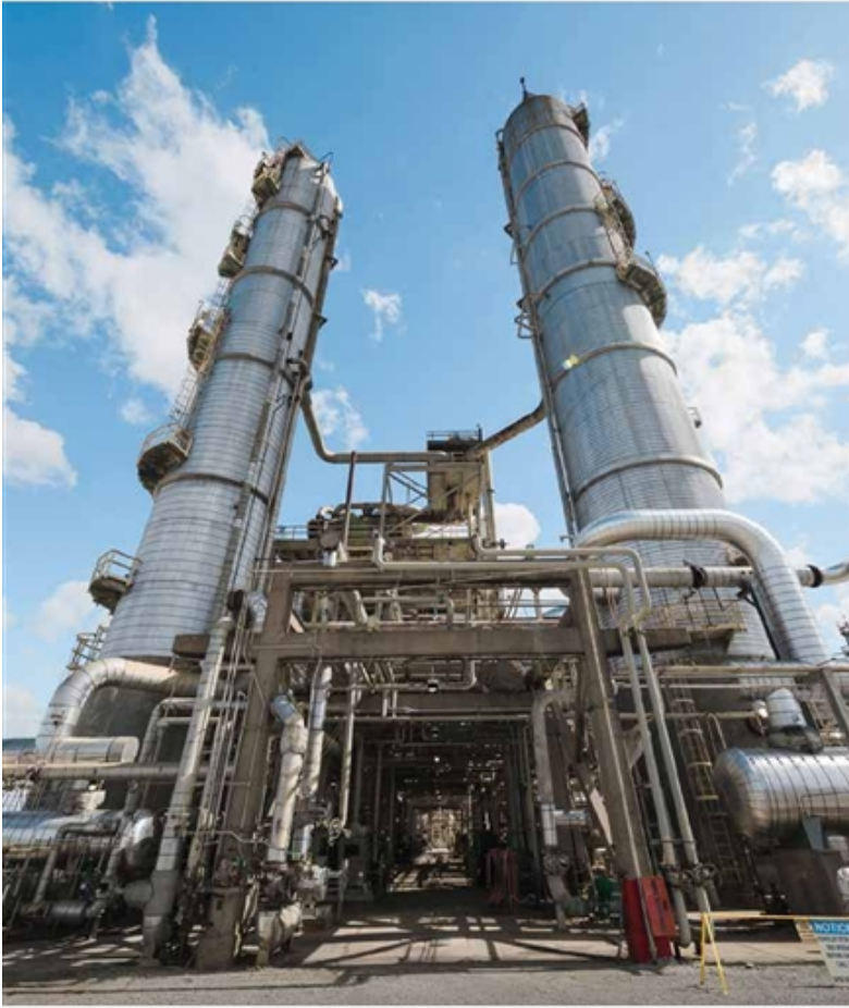
→ A chemical unit at ExxonMobil's Beaumont, Texas, facility.
