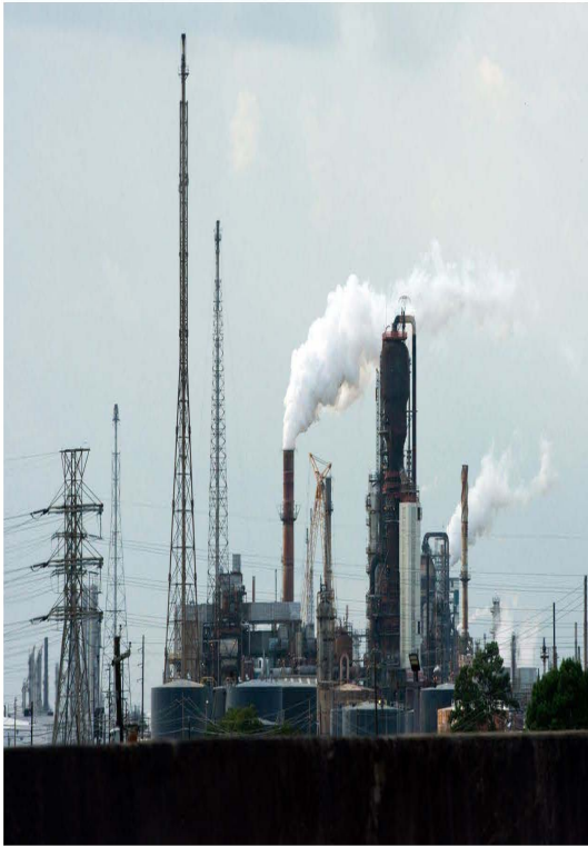
An Exxon Mobil plant in Baytown, Texas.
