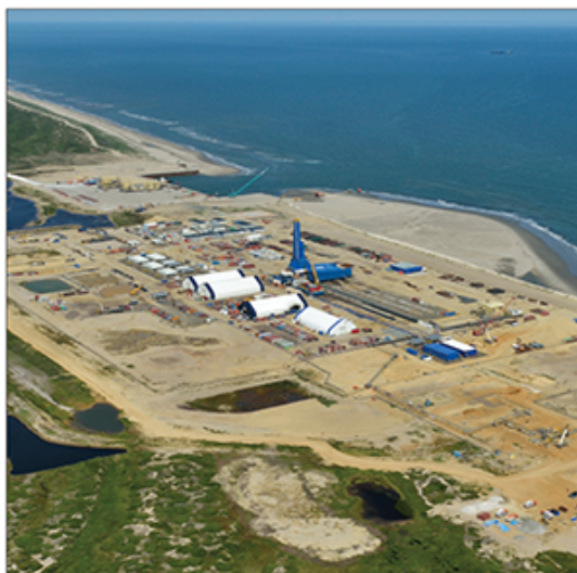
The Yastreb rig, Sakhalin Island, Russia, is one of the most powerful land rigs in the industry. In 2012, the rig drilled the world-record 7.7-mile-long horizontal well.
