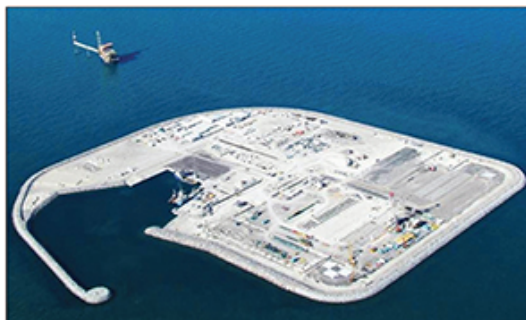
An innovative artificial island approach is being applied to efficiently gain access to new reserves at the Upper Zakum field in the United Arab Emirates.
