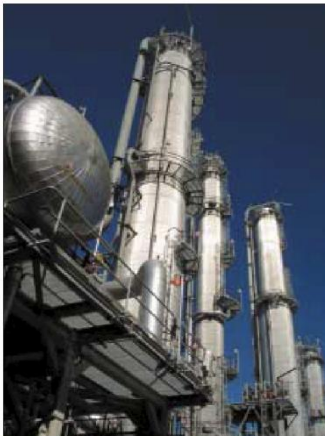
The Beaumont, Texas, aromatics facilities upgrade refinery feed streams to benzene and paraxylene using proprietary ExxonMobil technologies and catalysts. Refinery integration allows optimization of feed-and-return streams and lowers unit costs.
