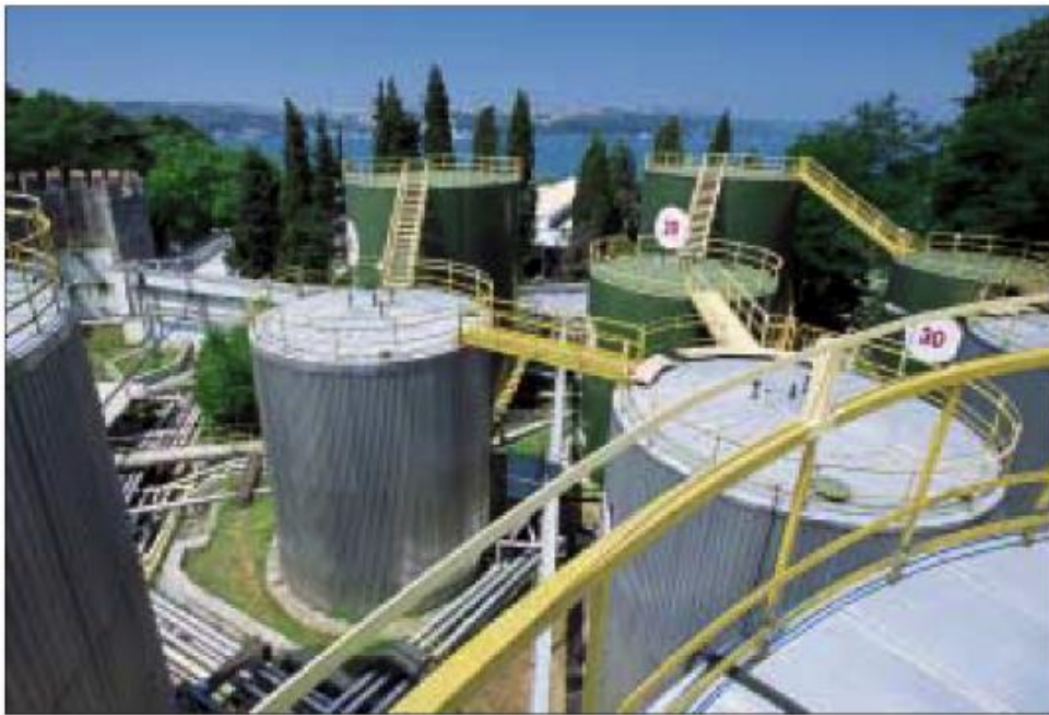
ExxonMobil's Servibernu Lube Oil Blending Plant in Istanbul, Turkey, is well positioned to meet demand growth in Turkey, Balkan states, and former Soviet Union countries.
