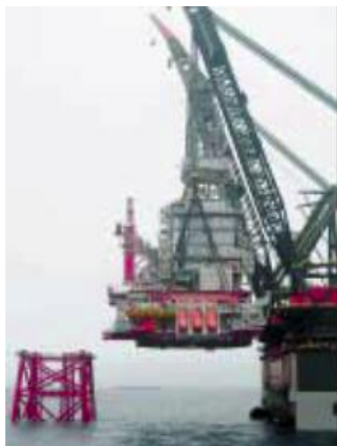
The Ringhorne platform in the Norwegian North Sea started production in early 2003. The topsides lift set an ExxonMobil record.
