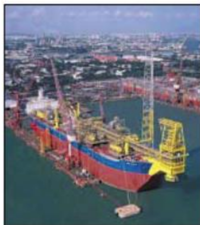
The Falcon FPSO vessel, during construction in Singapore, marks the first deployment of an Early Production System.
