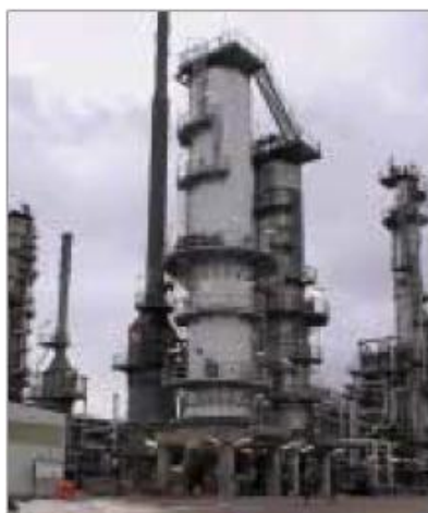
A new reactor started up in November, 2002, at the Slagen refinery in Norway for production of low-sulfur diesel fuel.
