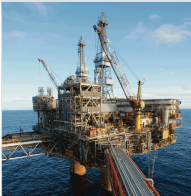
A new drilling program started at the North Sea Beryl field in 2009 that will develop additional reserves and extend field life.
