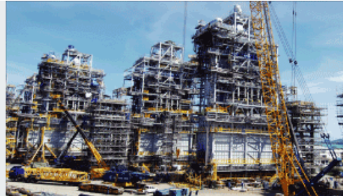
Proprietary technology to maximize feed flexibility is being built into these steam-cracking furnaces that will be installed as part of our Singapore expansion.
