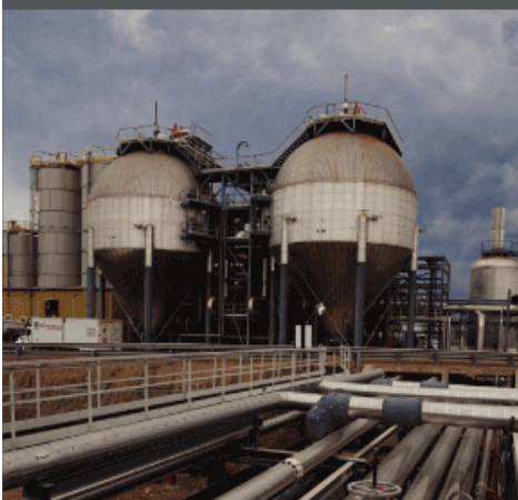
Water recycling units installed at the Cold Lake project in Canada allow 95 percent of the project's water to be reused.
