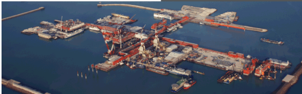
The Kashagan Phase 1 project uses artificial islands in the Caspian Sea to support drilling and production operations.
