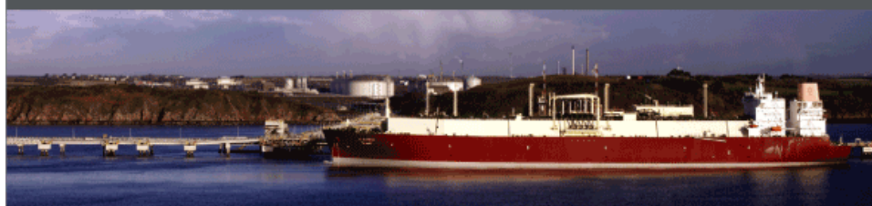
The South Hook LNG regasification terminal opened in 2009 and will have the capacity to deliver 2 billion cubic feet of gas per day. It will be supplied with LNG from Qatar's North Field using the world's largest carriers, including the Q-Max vessel Al Samriya pictured here.
