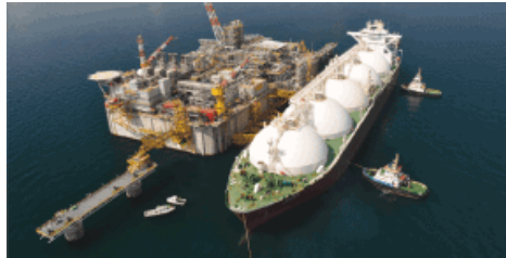
The Adriatic LNG Terminal is the world's first fixed offshore regasification facility and can supply about 10 percent of Italy's gas market needs. It received its first cargo in 2009.
