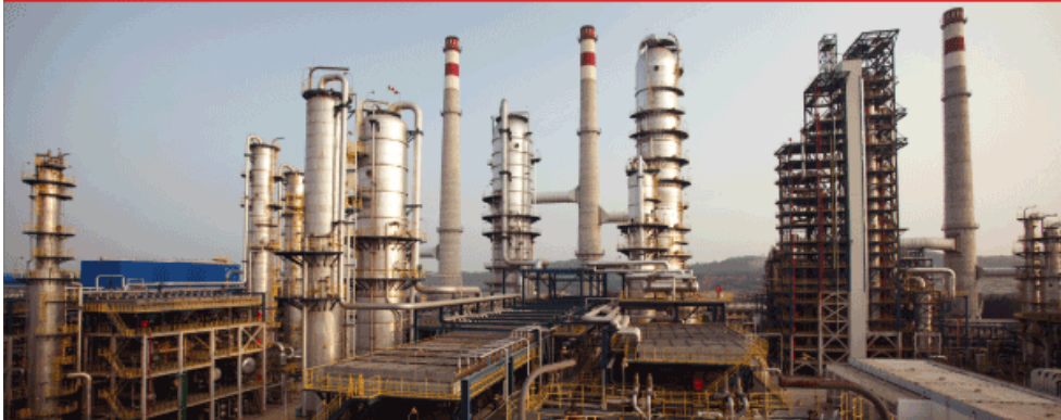
Start-up of the world-class petroleum refining and petrochemical complex in China's Fujian Province was completed in 2009. Included in the project was a tripling of refining capacity and an addition of two cogeneration units totaling 250 megawatts.
