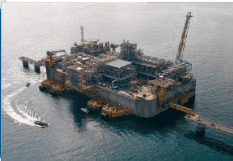
The Adriatic LNG Terminal can supply up to 775 million cubic feet of gas per day to the Italian market. It is the first gravity-based, fixed offshore LNG regasification terminal in the world.
