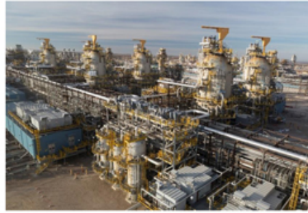
Heavy Oil Kearl Expansion
