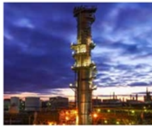
→ Concept of divided wall columns is applied to provide energy and capital savings by combining a series of distillation towers into one, as demonstrated at the Fawley Refinery xylene tower in the U.K. (picture shown above).
