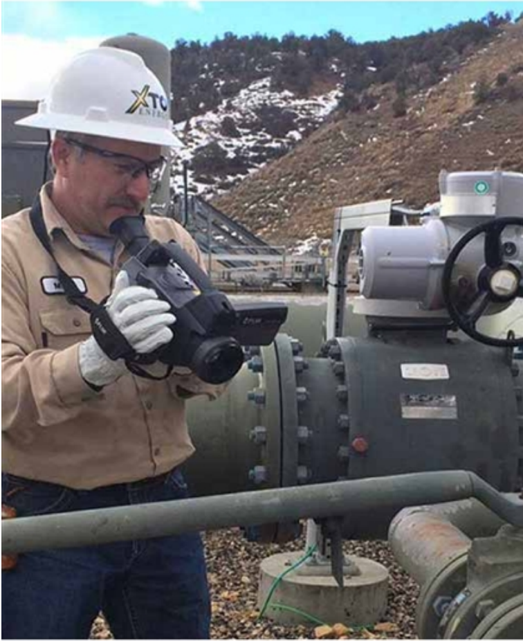
→ Leak-detection equipment is used to reduce methane emissions in Texas and New Mexico.
