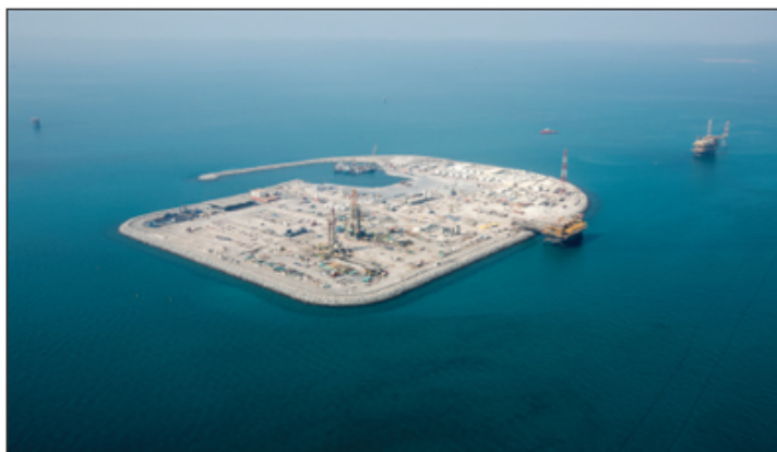
Drilling was initiated in 2014 from the artificial islands at Upper Zakum, United Arab Emirates, with plans to expand production to 750 thousand barrels per day.
