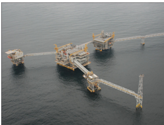
Natural gas liquids are produced from the East Area Complex in Nigeria.
