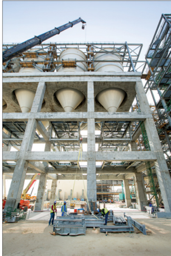
In 2014, we progressed construction on facilities in Al-Jubail, Saudi Arabia, that will produce a broad range of synthetic rubber and related products.
