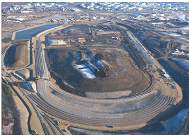
The Edmonton Rail Terminal will have a capacity of 210 thousand barrels per day, enabling us to efficiently export equity crude from Western Canada.
