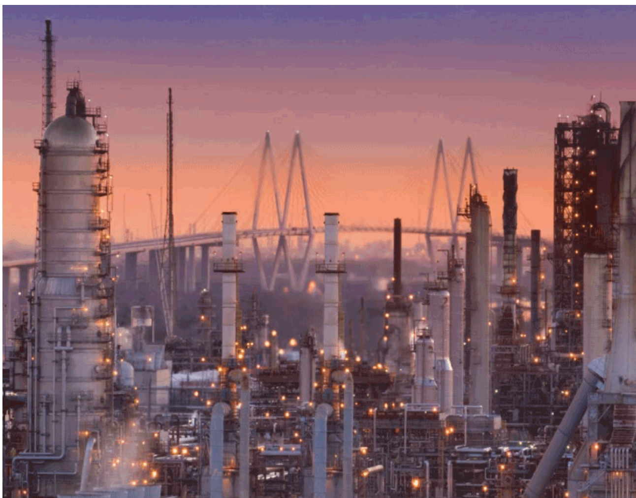
ExxonMobil's Baytown, Texas, refinery is the largest in the United States, with capacity to process over 560 thousand barrels per day of crude oil into low-sulfur gasoline and diesel, chemical feedstocks, lubricants, specialties, and other petroleum products.
