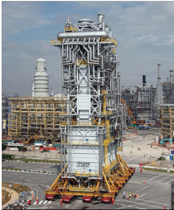
As part of the Singapore expansion project, seven steam-cracking furnaces have been installed (one shown above in transit). These furnaces are the largest of their kind: each weighs the equivalent of five jumbo commercial airplanes and is 15 stories tall. They employ our state-of-the-art, proprietary technology and are part of a feed-flexible steam cracker that will add 1 million tonnes per year of ethylene capacity.
