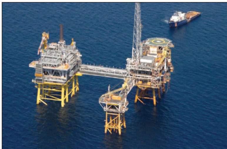
The Sable platforms connect five offshore gas fields that supply energy to markets in eastern Canada and the northeastern United States.
