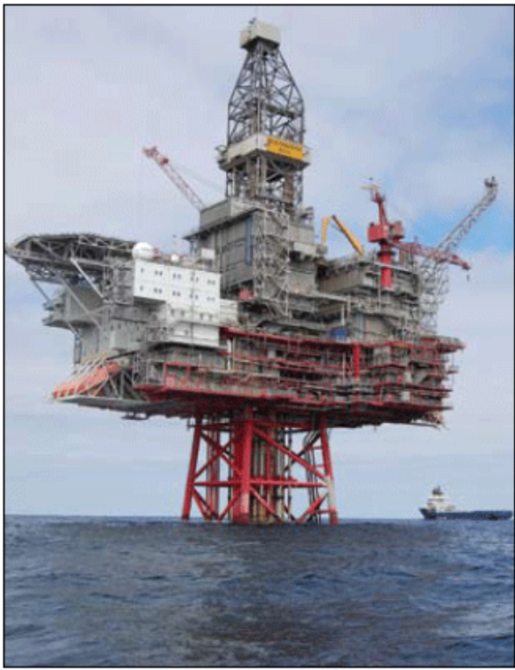
The ExxonMobil-operated Ringhorne platform is 110 miles offshore Norway in 410 feet of water.
