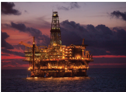
Angola Block 15 facilities, including the asset at Kizomba B, continue to operate with very high reliability.
