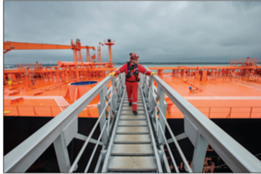
Shared site management, support services, utilities, and infrastructure lead to lower cost at integrated refining, chemical, and lubricant manufacturing complexes such as our Fawley Refinery.
