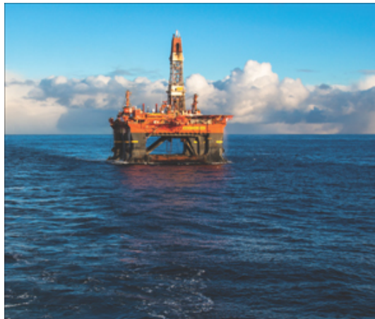
The West Alpha Rig, in Norway, commenced drilling at Balder in February 2013.
