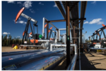
Steam Injection Cold Lake Nabiye
