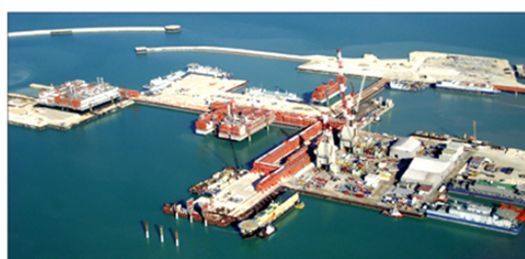
Artificial islands in the Caspian Sea support the offshore drilling and production activities for the Kashagan Phase 1 development.
