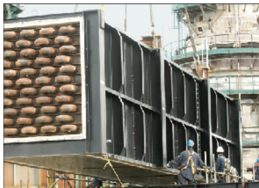
A new furnace is installed in the vacuum distillation unit of the Dartmouth refinery in Nova Scotia, Canada. This project will increase capacity and reduce energy usage.
