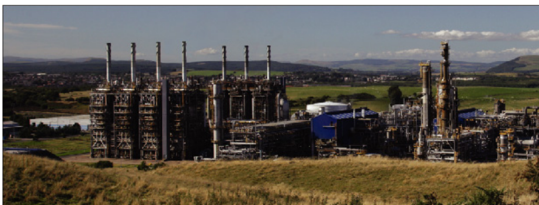
Steam cracking remains the foundation of the petrochemical industry. The Fife Ethylene Plant in the United Kingdom is one of Europe's largest and most modern steam crackers, producing ethylene from North Sea natural gas liquids.
