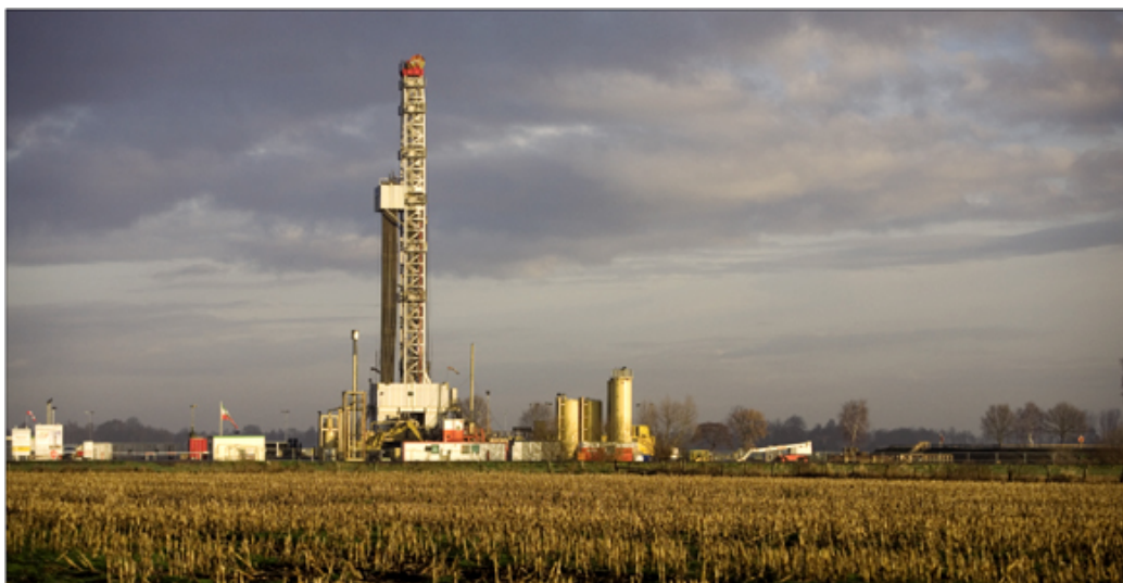
Drilling activities are under way in the Lower Saxony Basin, Germany, to explore for unconventional gas resources to help increase natural gas supplies in Europe.
