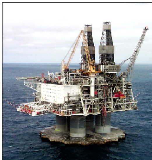
The Hibernia platform offshore Newfoundland, Canada, can store 1.3 million barrels of oil in its gravity-based structure.
