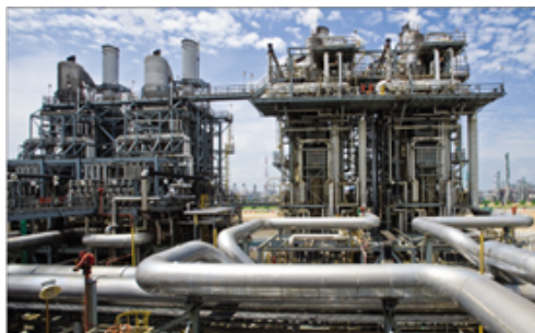
The Singapore Chemical Plant is fully integrated with ExxonMobil's largest refinery. The addition of a second world-scale petrochemical facility in Singapore will help meet increasing demand in Asia and reinforces ExxonMobil's commitment to the petrochemical business.
