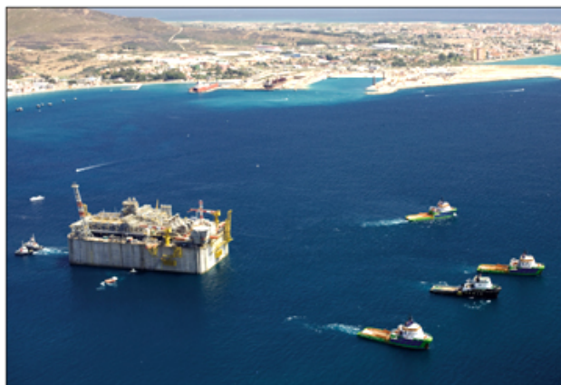
The Adriatic LNG terminal was towed from its construction site in Algeciras, Spain, to its final destination offshore Porto Levante, Italy. Commissioning activities are under way for start-up in 2009.
